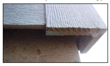
This often leads to water absorption and eventual swelling. Therefore, I suggest adding primer and paint to the bottom edges of all siding and trim adjacent to the foundation and around windows to help protect against water damage.
