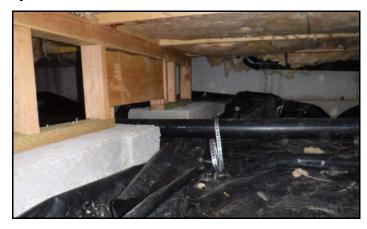
11. I found two sections of interior footing curbs in the crawlspaces under the front entry with no pony wall supports, as shown in the following photo. Occasionally, I find footing curbs in the crawlspaces that are not part of the original blue prints, and were poured needlessly. However, I suggest verifying with the builder/framing contractor whether or not pony wall intermediate supports are necessary at this location.
