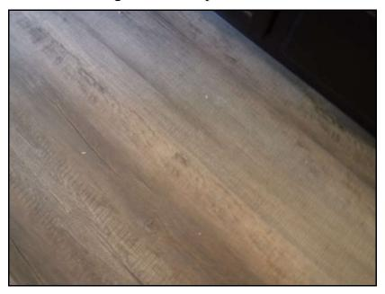
p. I found specks of ink splatter on the attic side of the OSB roof sheathing, as exemplified in the following two photos. This occurs during manufacture, and is strictly cosmetic. (Some people may erroneously mistake these splatters as biogrowths.)
