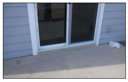
This can encourage moisture to wick up into the trim, which can lead to possible deterioration. Siding and trim should be held at least 1 inch above concrete to help prevent such issues. Furthermore, the materials behind and below the siding and trim should be protected with flashing designed and installed to effectively prevent water entry behind the concrete.
