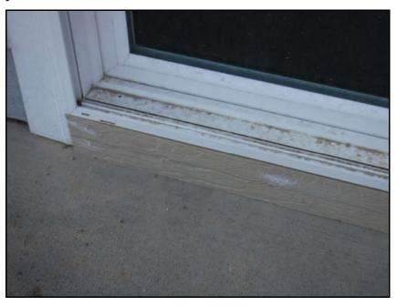
7. Some of the caulking is starting to split along the seams of the siding and trim around the home, as exemplified in the following photo. This can eventually allow water entry resulting in swelling.
