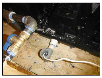
• The HVAC system in the attic drains into an open attic drain beneath the furnace, as shown in the following photo. It has a water trap and should stay wet year-round if heated and cooled. However, any potential clogs or backups could allow moisture to overflow into the attic.
