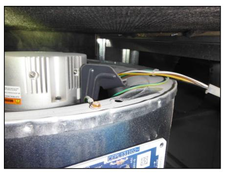
21. The viewing glass panel is missing through the blower compartment cover of the furnace in the attic, as shown in the following photo. This can allow attic interior air to be pulled through the blower during operation of the furnace.
