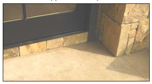
5. The masonry on the support posts at the rear exterior are in contact with the adjacent concrete, as exemplified in the following photo. This can encourage moisture wicking and potential cracking of the mortar or masonry during potential seasonal or intermittent frost heaving.
