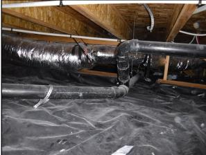
These straps should be securely in place at least every 4 feet to adequately support the horizontal runs of the drain piping in order to help eliminate sags that could eventually trap solids and cause blockages. (The horizontal runs of drain piping should always slope between ¼ and ½ inch per foot towards the collection system.)
