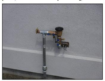
The purpose of this valve assembly is to protect public drinking water systems (including aquifers) from possible cross contamination that could seriously threaten public health. Please understand that there is no "grandfathering" of older valves where public safety is at risk. (NOTE: Although state code requires annual reinspection of these valves by certified backflow prevention inspectors, many property owners are still unaware of this law and have water systems out of compliance.)
