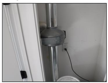
The exhaust fan should cost only pennies per month to run, and should operate very quietly. Such fans are purposely sized to draw only reasonable amounts fresh air into the house without having to pay too much to either re-heat or re-cool the living spaces because of the incoming fresh air.
