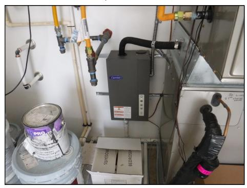
• After running the air conditioner for more than 10 minutes, I measured a cooling effect differential of 19 F° between feed-air and return-air registers close to the air handler, as shown in the following photos. (Cooling effects outside the range of 17 to 22 degrees are usually considered "problematic" and warrant the attention of a licensed HVAC contractor.)
